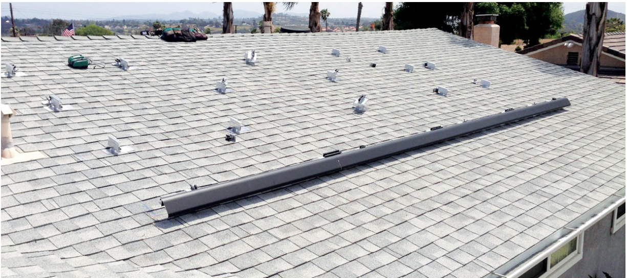
ABOVE: Roof mounts and skirting installed for a railless mounting system. The skirting is optional and provides a finished look to the most visible portion of the array.
