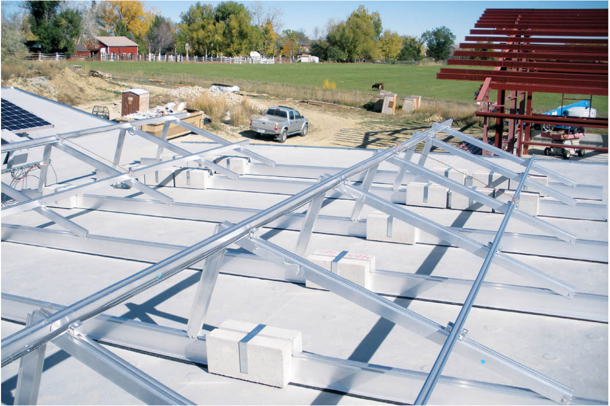
ABOVE: Flat-roof system with horizontal base rails weighted with concrete blocks (ballast)
