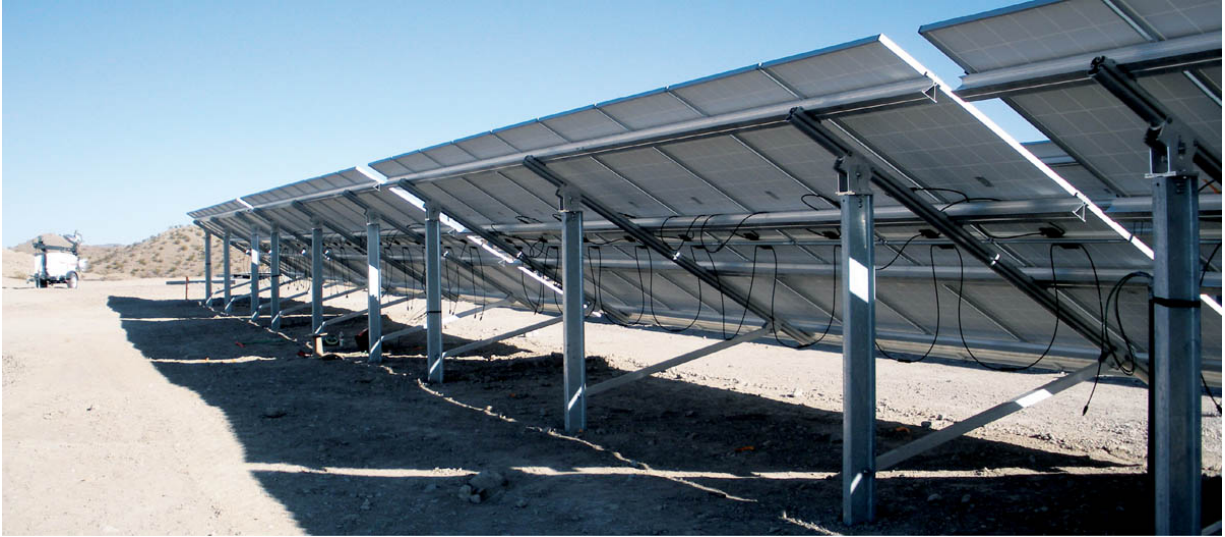
ABOVE: Standard ground-mount, single-post, cantilever design
