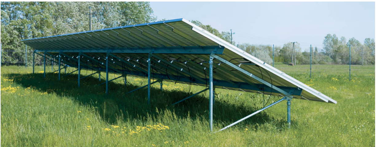
ABOVE: Standard ground-mount with two rows of vertical posts
